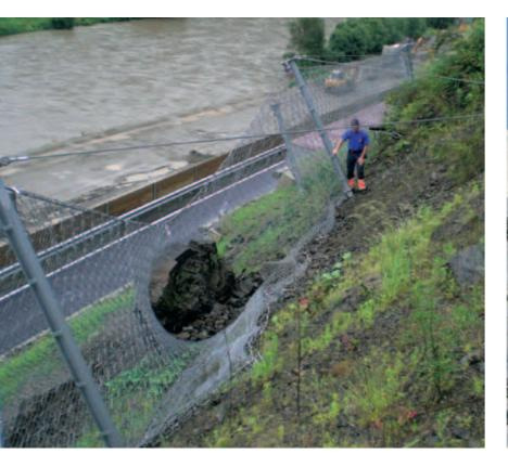
Rockfall protection systems or catchment fences serve as secondary protection from falling and sliding rock in potential run-out zones or areas of deposition. They are used for the protection of inhabited areas and infrastructure.
