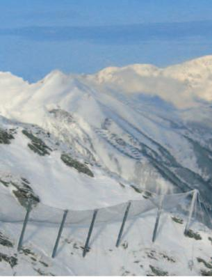
The avalanche protection systems by Trumer Schutzbauten utilize the flexible nature and high strength of the Omega-Net to prevent avalanches in their first stage of occurrence. This means the hazard is essentially removed prior to the start of an avalanche and not just mitigated once it has occurred.
