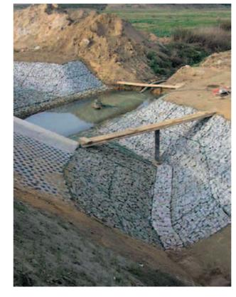
Weldmesh Mattresses are prefabricated from welded steel wire mesh. Mattresses are manufactured from lighter grades of wire to increase their flexibility.
