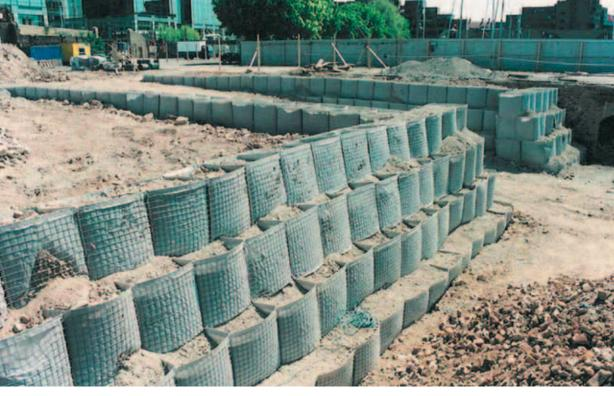
Betafence Weldmesh® Gabions are wire mesh baskets formed by connecting individual panels of mesh with helical spirals on the vertical edge wires creating an open series of box compartments that fold in a concertina fashion to be flat packed. Lids and bases are sometimes supplied loose with helical spiral binders to connect the top and bottom of the open cells along one edge. Alternatively they may be factory fitted where practical for ease of transportation.
