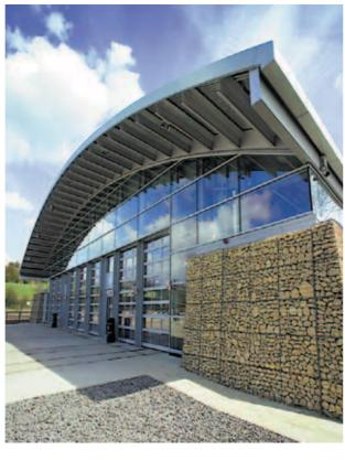
Betafence Weldmesh® Trapions are a form of Gabion manufactured from welded wire mesh panels with either one or both faces inclined at varying angles to the horizontal dependant upon the unit's height. They are supplied in lengths of 1, 2 or 3m or part lengths thereof, and pre-assembled with helical spirals for flat packing and ease of transportation to site.
